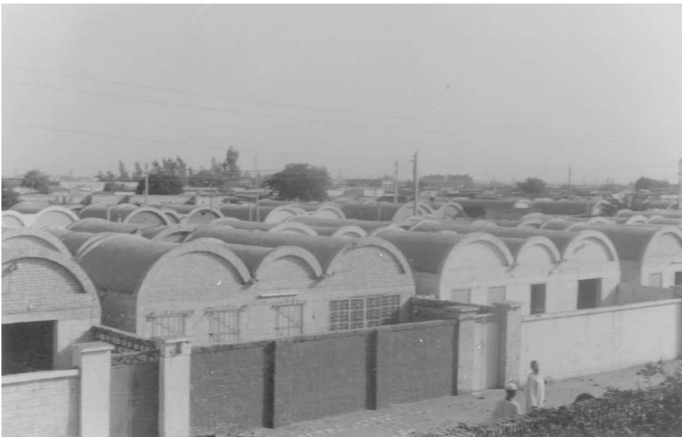
Photo 2. A view of Hai Al-Hajar (As-Souq Ash-Sha c bi) housing showing the designer's attempt to reduce construction costs and create character through the use of brick vaults.
